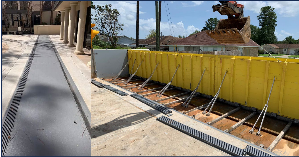
Figure 19: Passive flood barrier shown in passive state (left) and deployed state (right) (Source: www.floodbreak.com )
