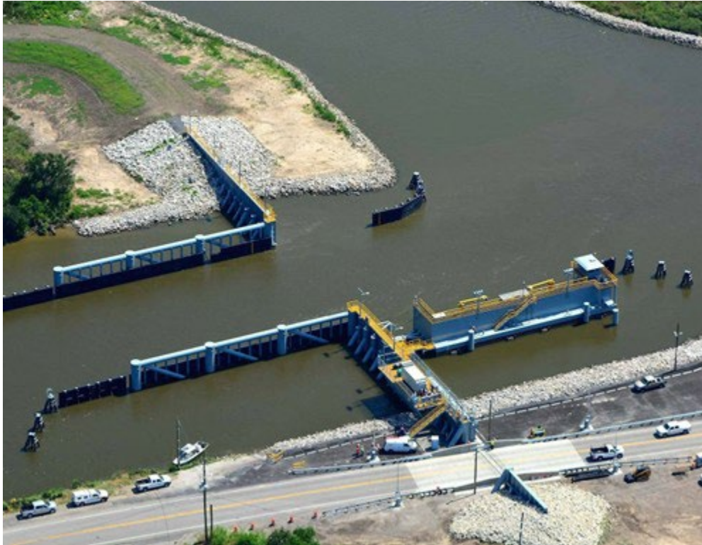
Figure 31: Barge Gate Example (Source: Terrebonne Levee & Conservation District, https://www.facebook.com/TerrebonneLevee/ )
