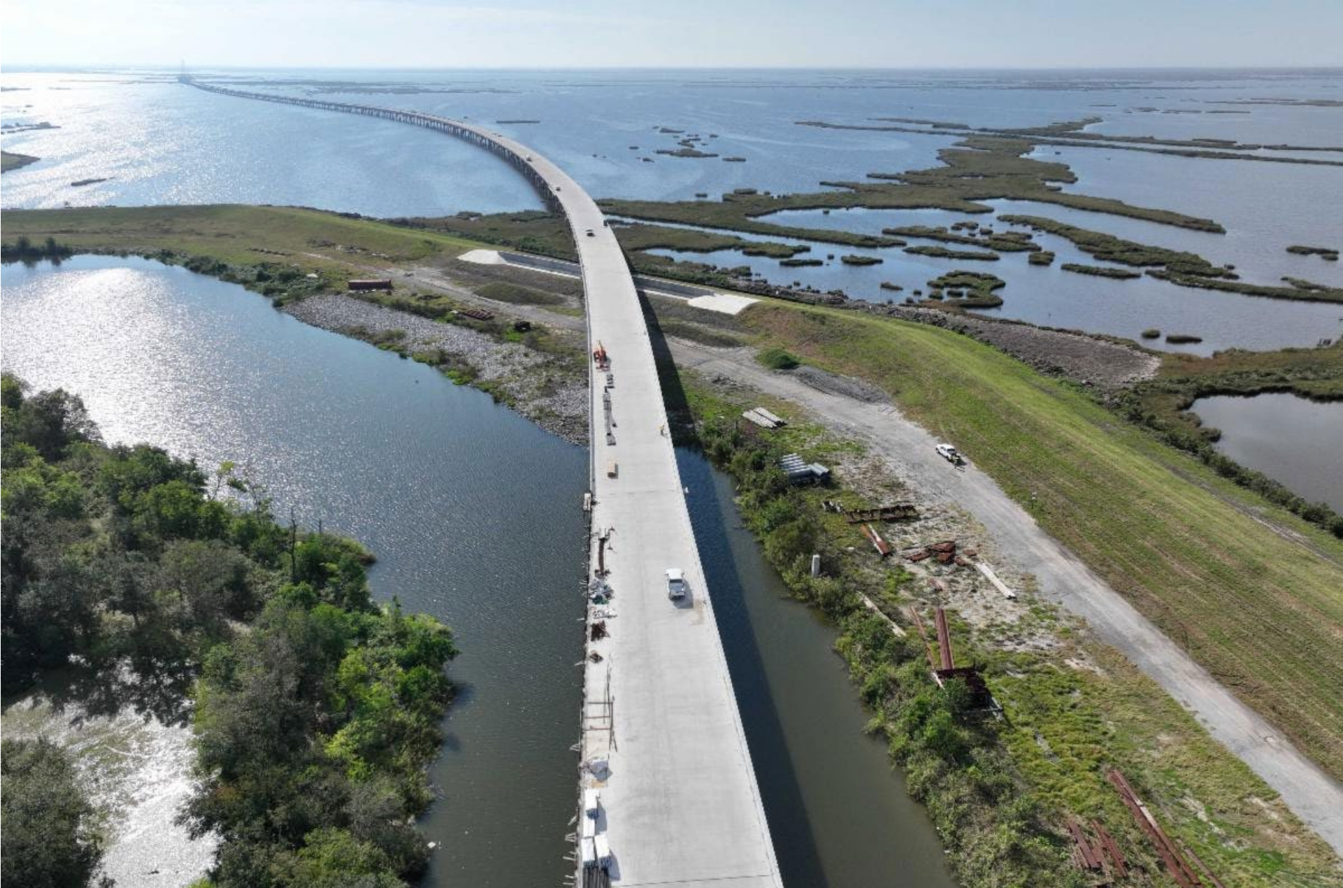
LA 1 crosses over South Lafourche Levee
