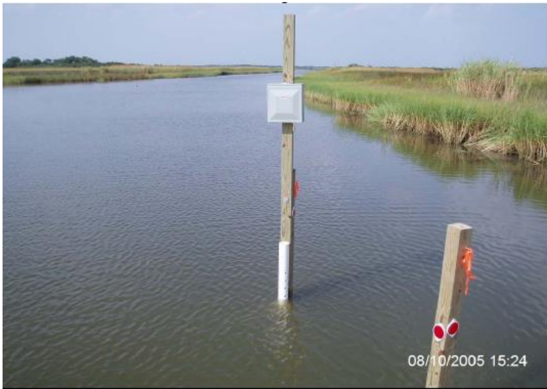
Figure A-3. Continuous recorder site (pvc and electrical box) in open water environment. Orange flagging represents the “nail” or TBM to be surveyed.
