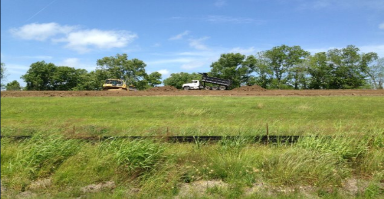
St. Gabriel Levee Enlargement Iberville Parish, completed in 2018
