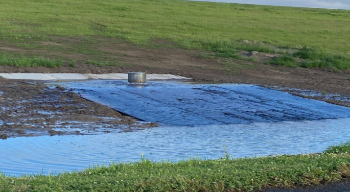
Upper Pontchartrain Seepage Control East Baton Rouge Parish, completed in 2024
