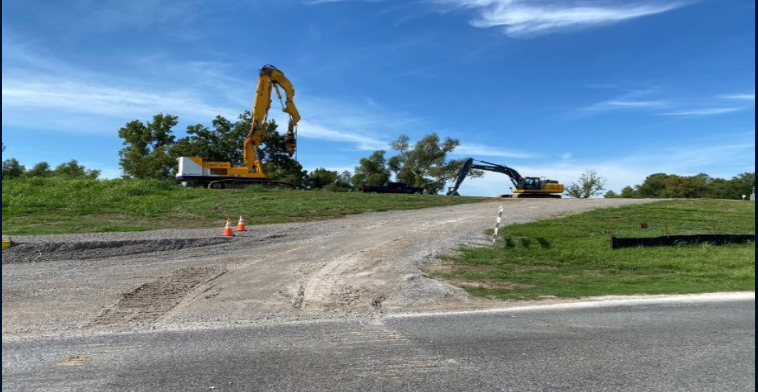
Plaquemine Point Seepage Control Iberville Parish, completed in 2025
