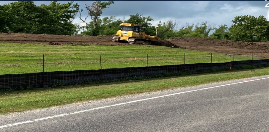
St. Rose Levee Enlargement St. Charles Parish, under construction
