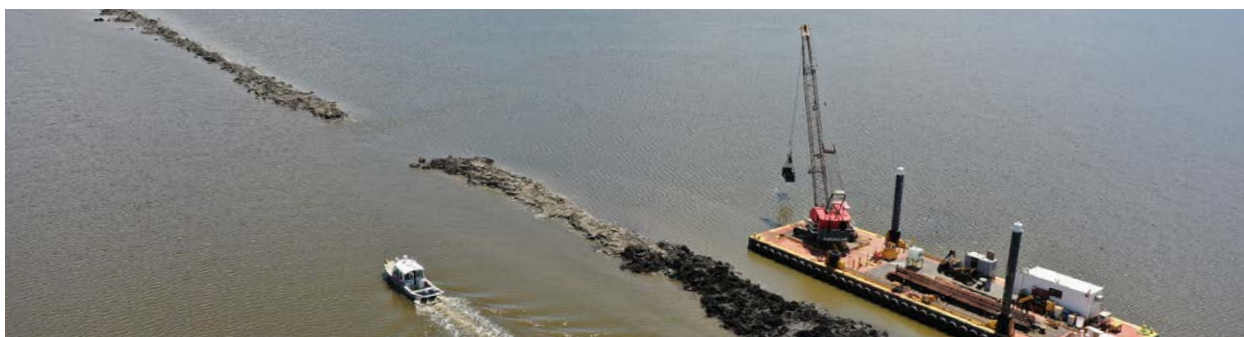
Ridge construction at Bayou Grand Cheniere in the Barataria Basin
