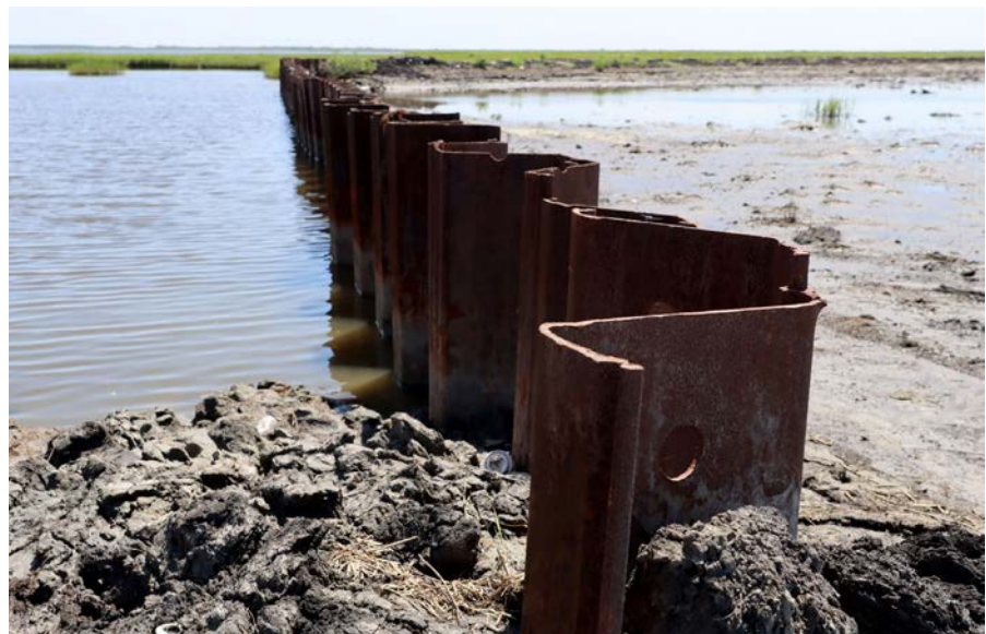
Sheetpile and dikes built for containment cells
