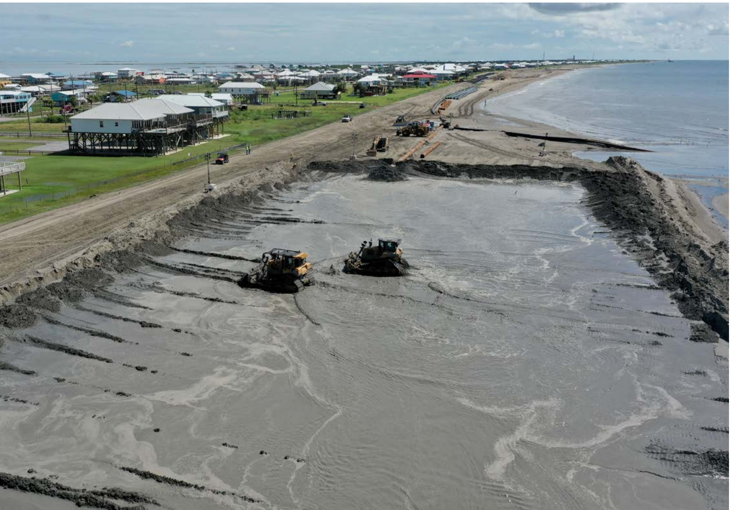
Grand Isle Dune and Beach Restoration
