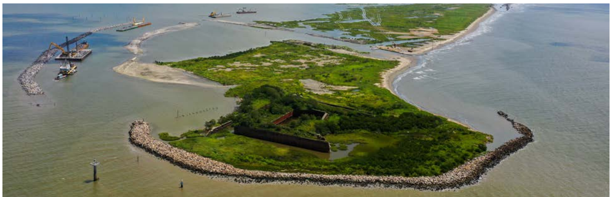
Newly fortified shoreline near Fort Livingston on West Grande Terre island
