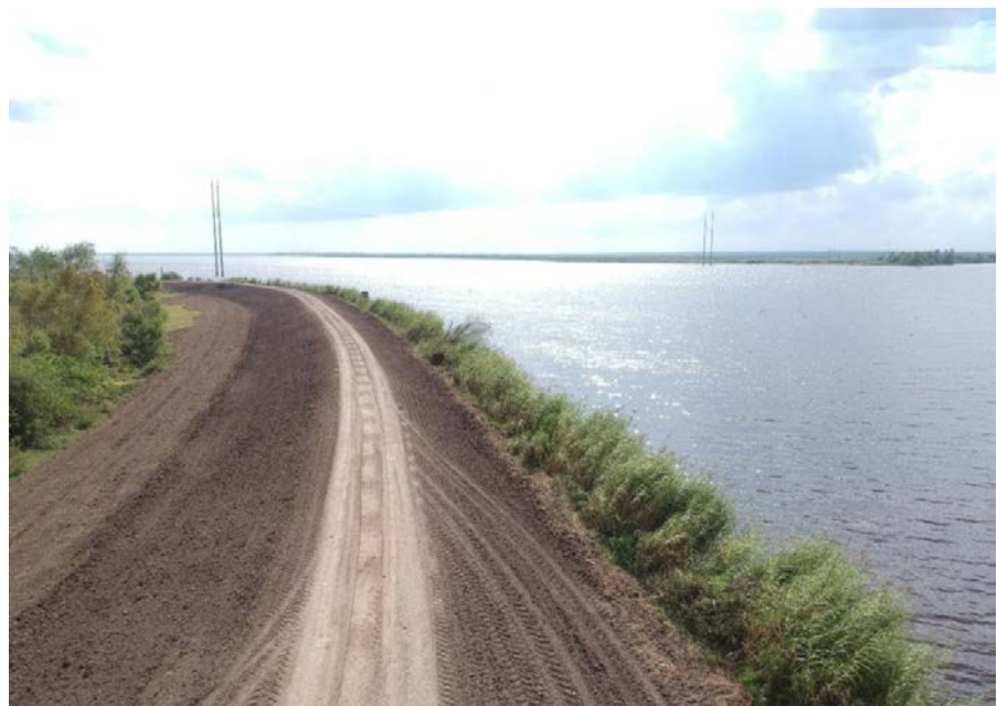
Newly constructed Sunset levee
