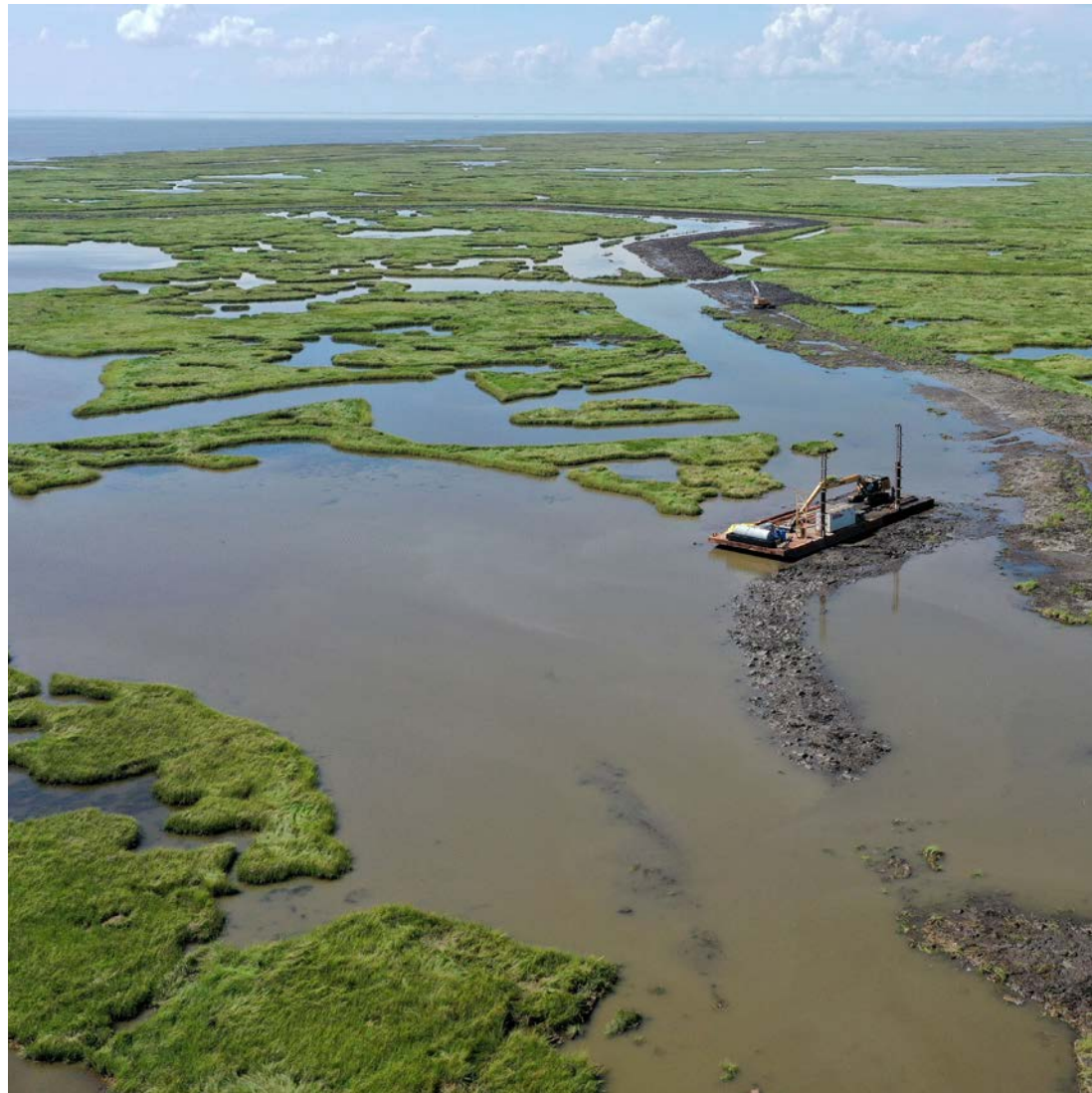
Dredging activity near Lake Borgne
