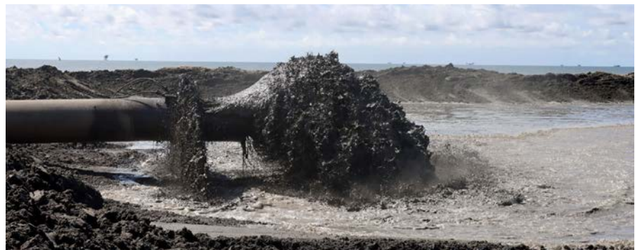
Dredge pipes pump material from the Gulf of Mexico to Grand Isle beach
