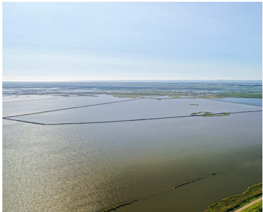
Containment dikes near No Name Bayou
