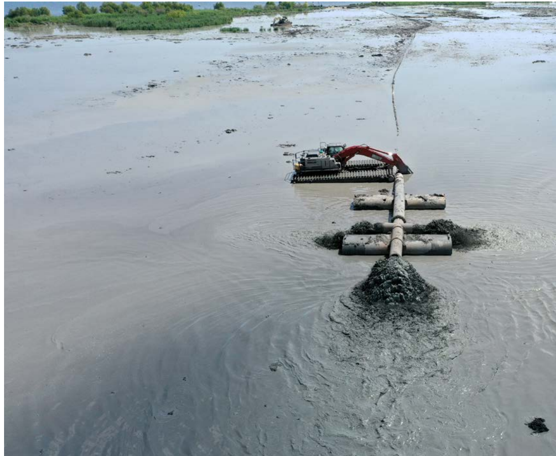
Dredging activity to restore the Labranche wetlands area
