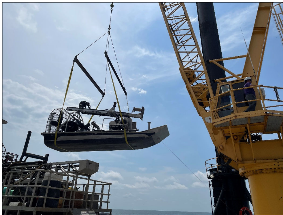
Figure 1: Airboat drill being lifted from the liftboat to the water.
