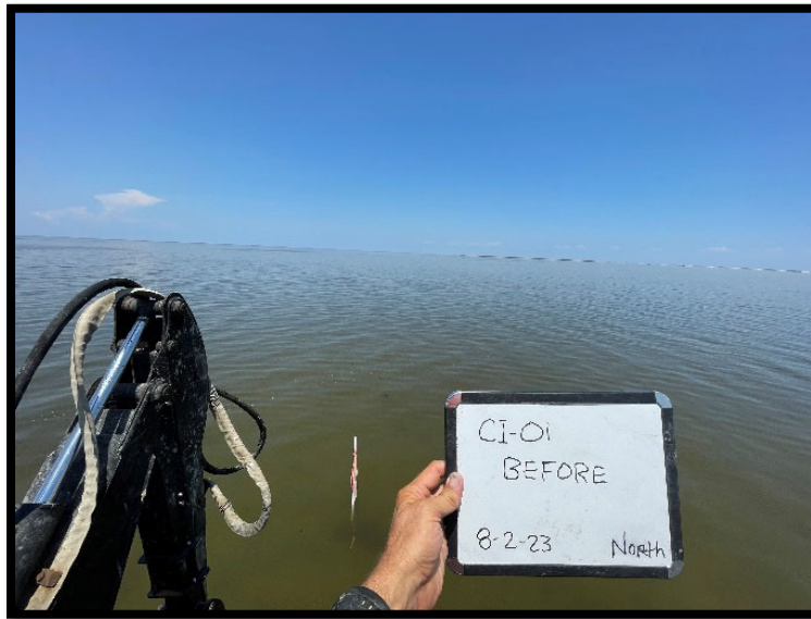
Figure 3: Boring CI-01 Site Conditions Before Drilling
