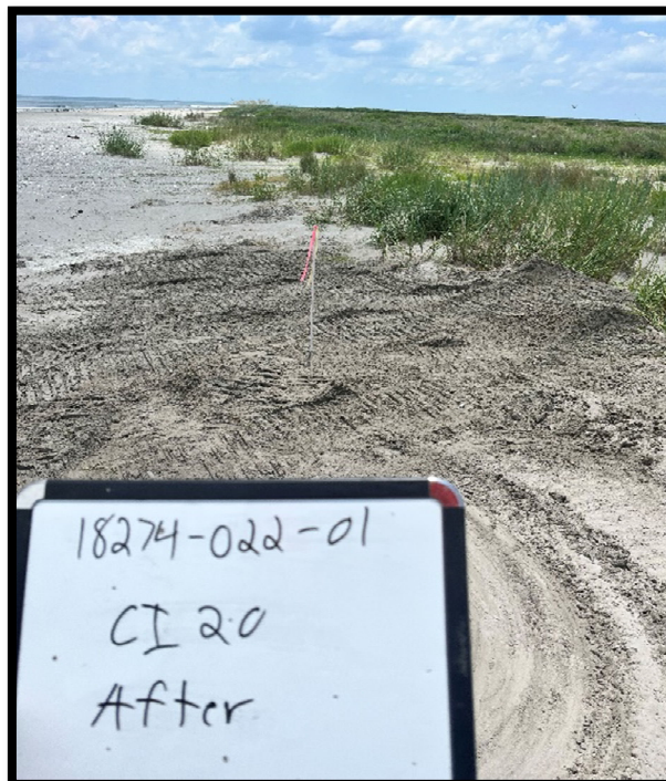
Figure 2: Boring CI-20 Site Condition After Drilling
