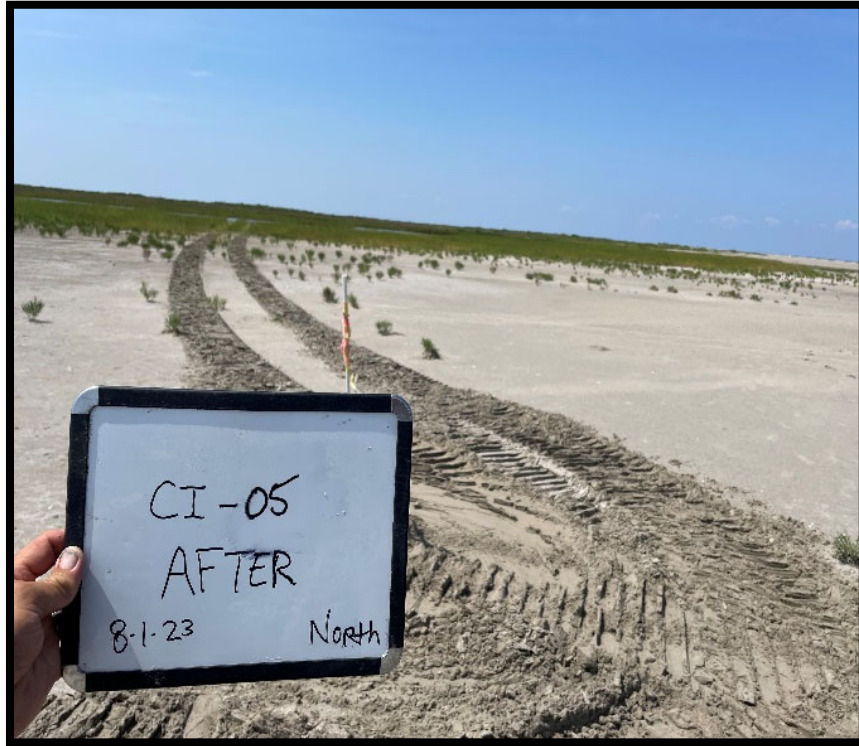
Figure 3: Boring CI-05 Site Condition Drilling
