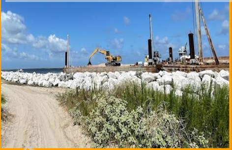
West Jetty Repairs
