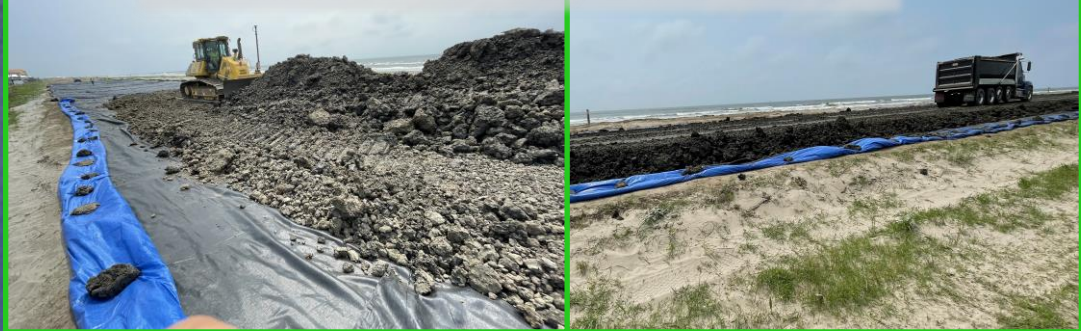
Construction of Clay Dune Cores
