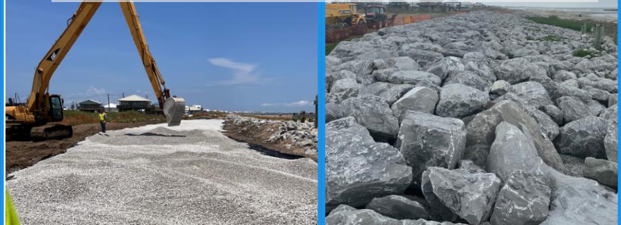
Construction of Stone Dune Cores
