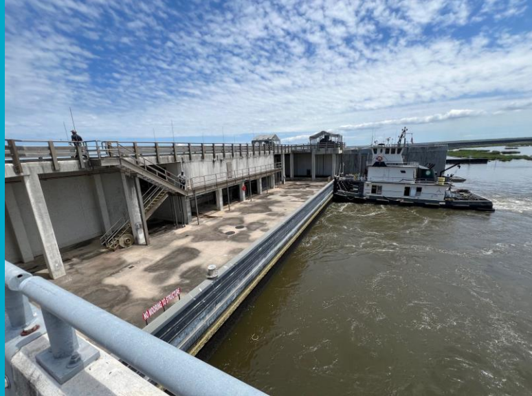
Surge Barrier Barge Gate Open and Closed Positions Closed for Hurricane Season – April 2024
