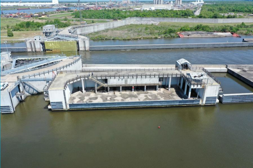
Surge Barrier Barge Gate Open and Closed Positions Closed for Hurricane Season – April 2024
