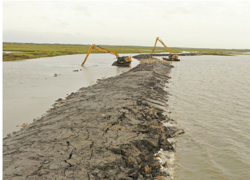
GRADING AND SHAPING
