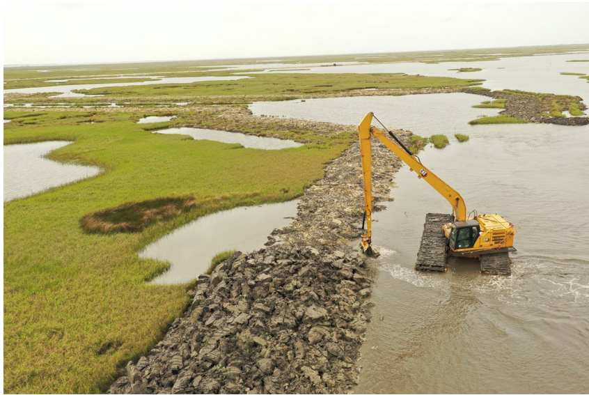
FIRST AND SECOND LIFTS
