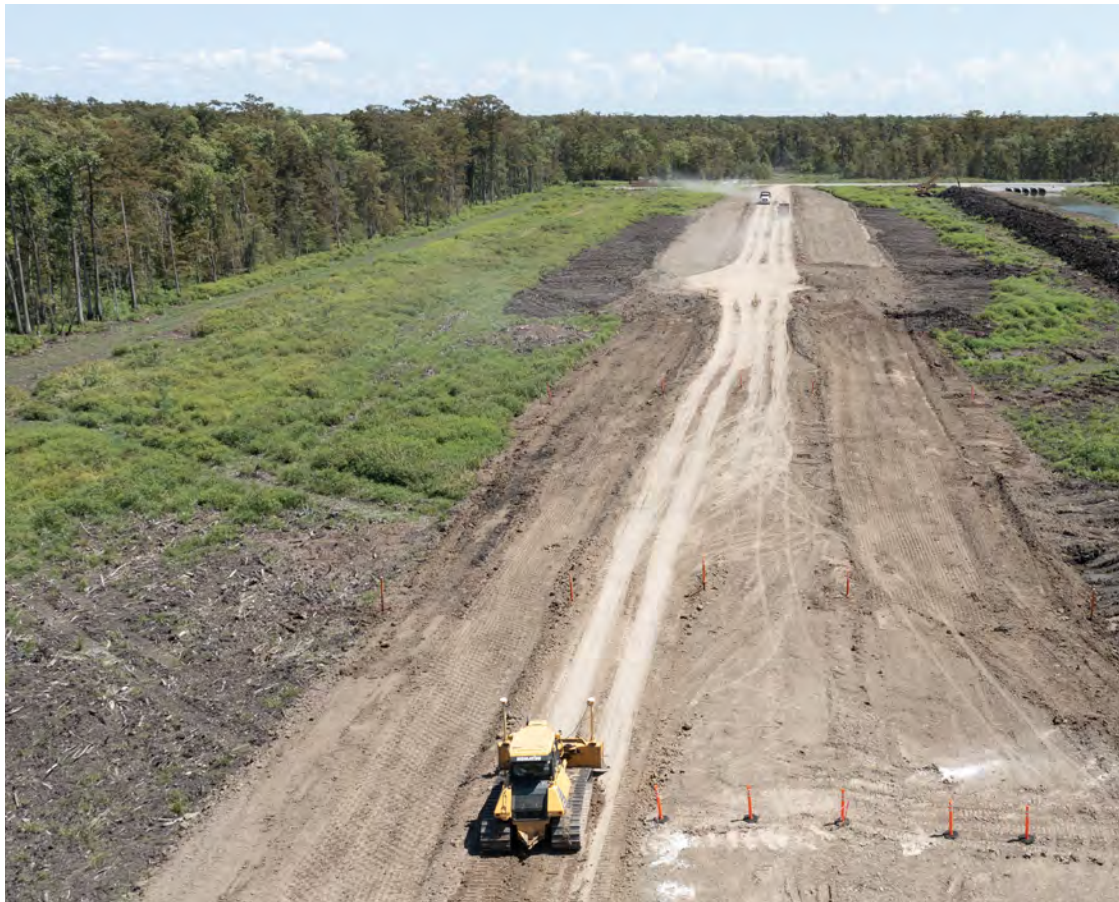
Earthen levee construction on the WSLP levee system
