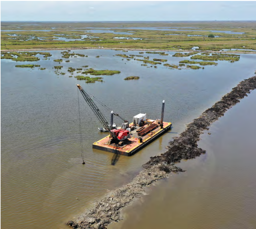
Containment dike construction at Bayou Grande Cheniere
