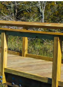
Cypremort Point Marsh Boardwalk
