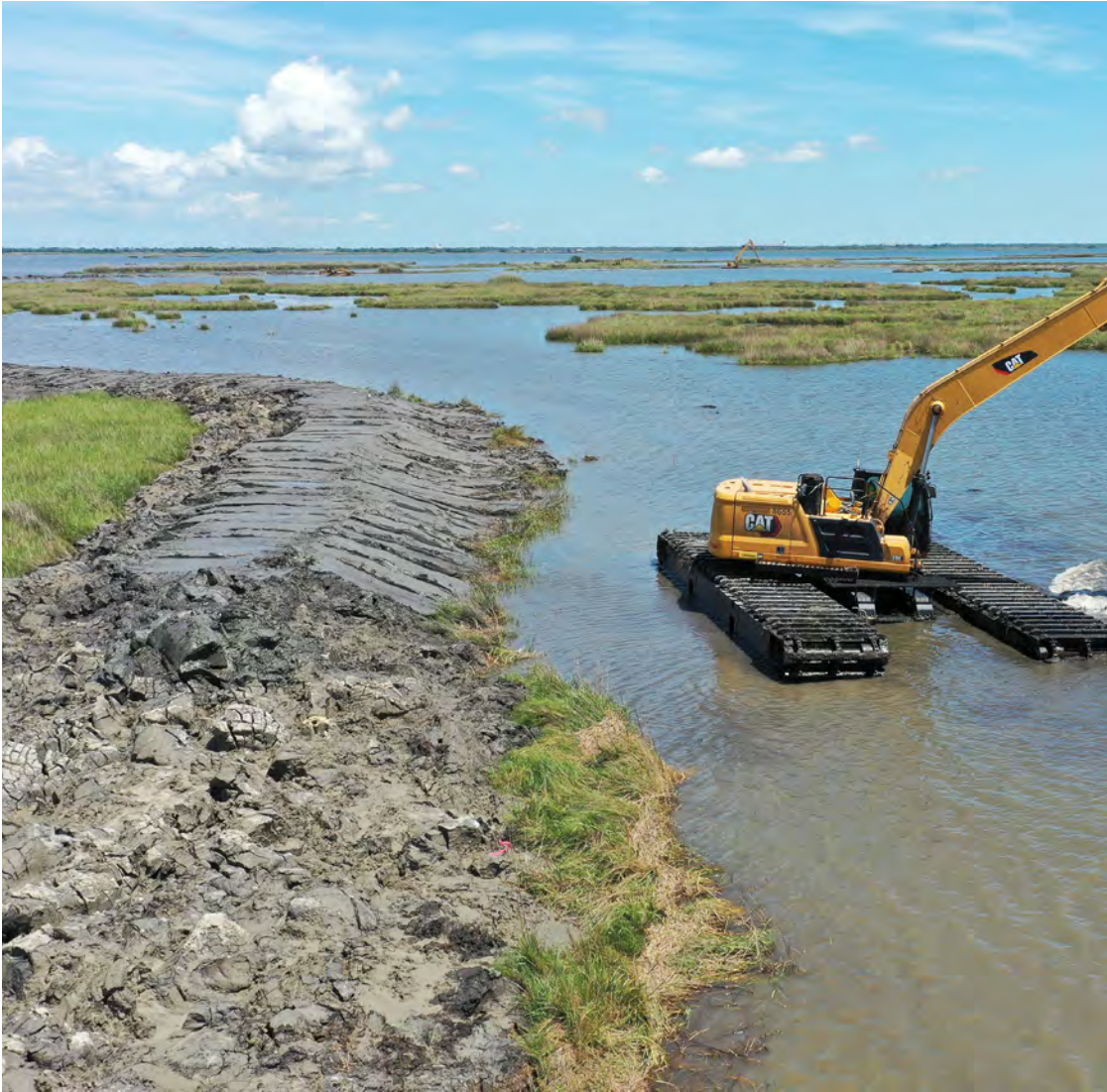
Construction on the Bayou Grande Cheniere Marsh Creation project
