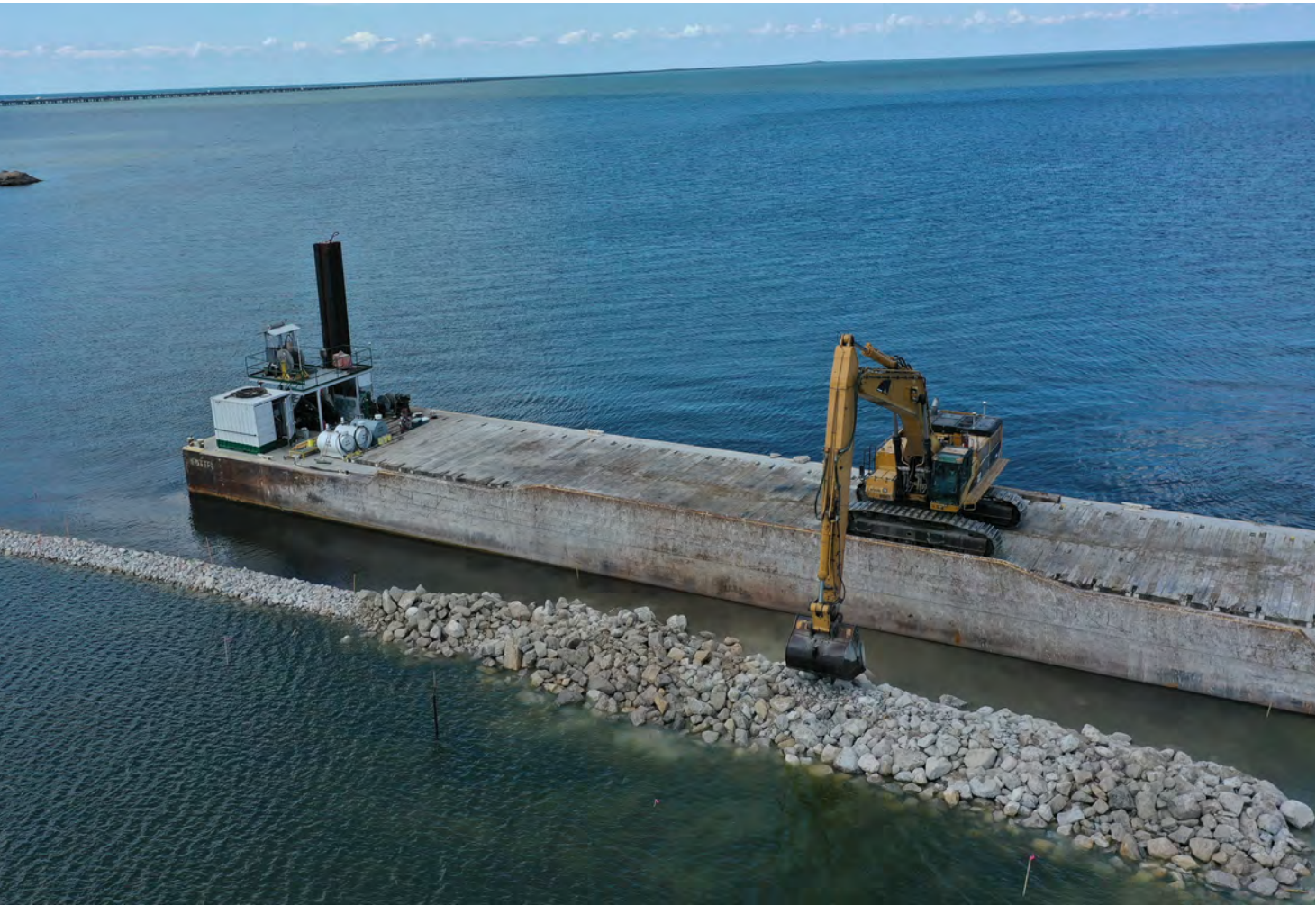
Bucktown Living Shoreline Construction
