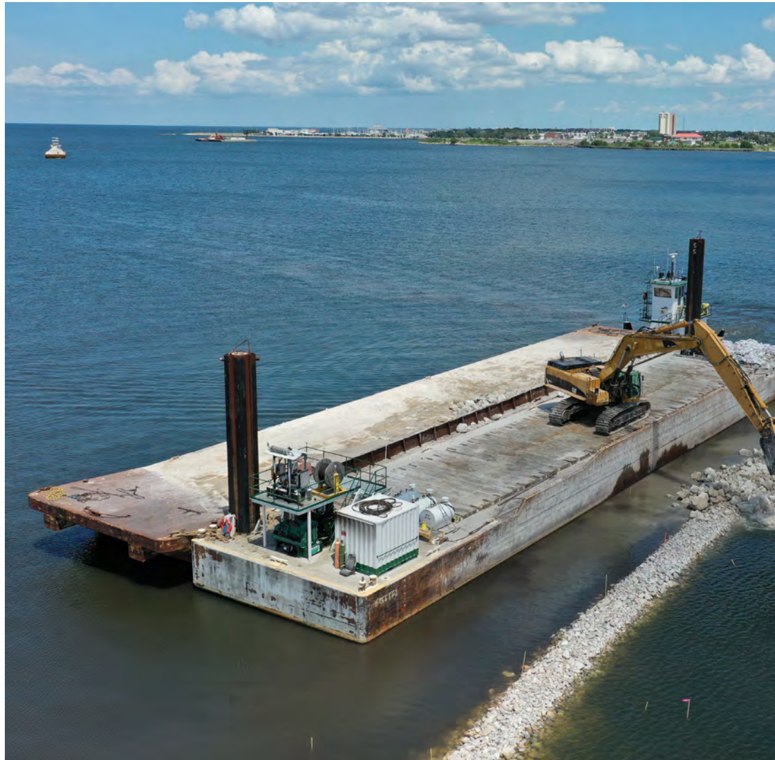
Construction begins on the Bucktown Living Shoreline
