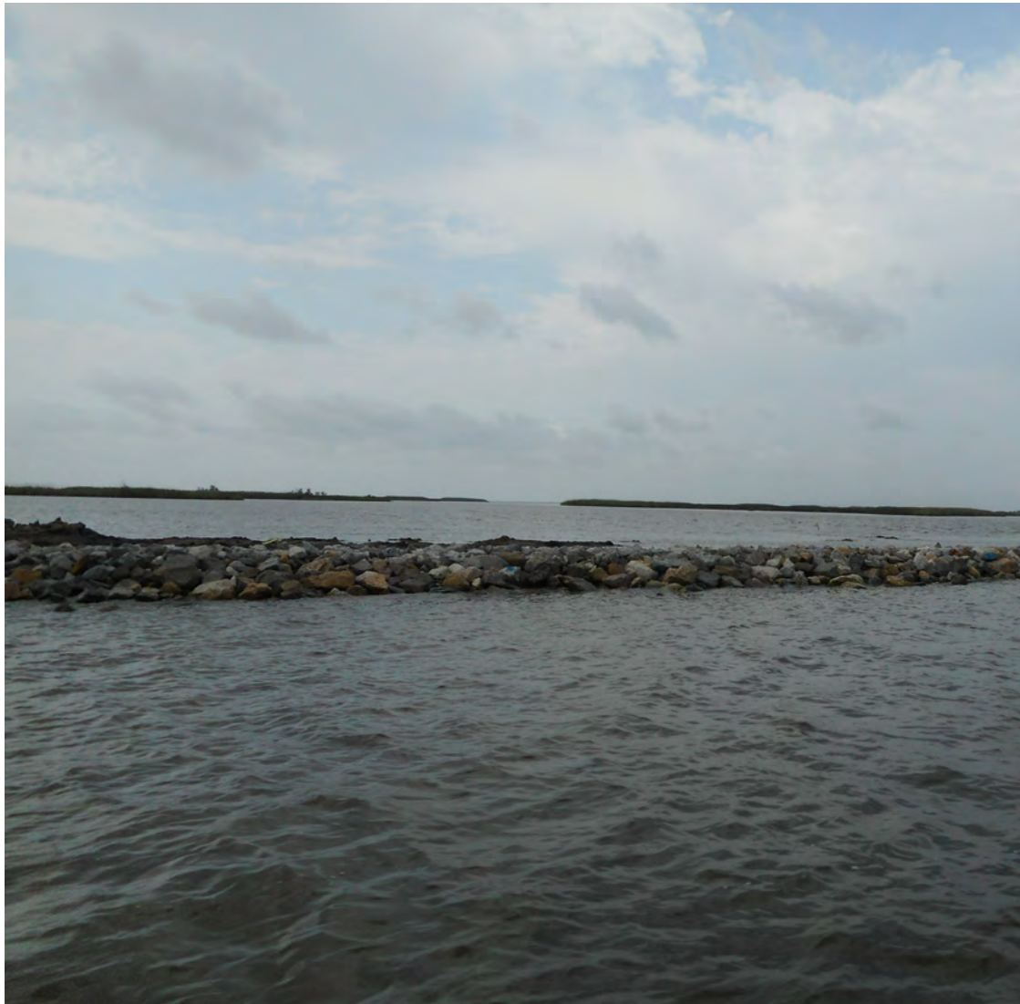
Freshwater Bayou Shoreline Protection project upon completion
