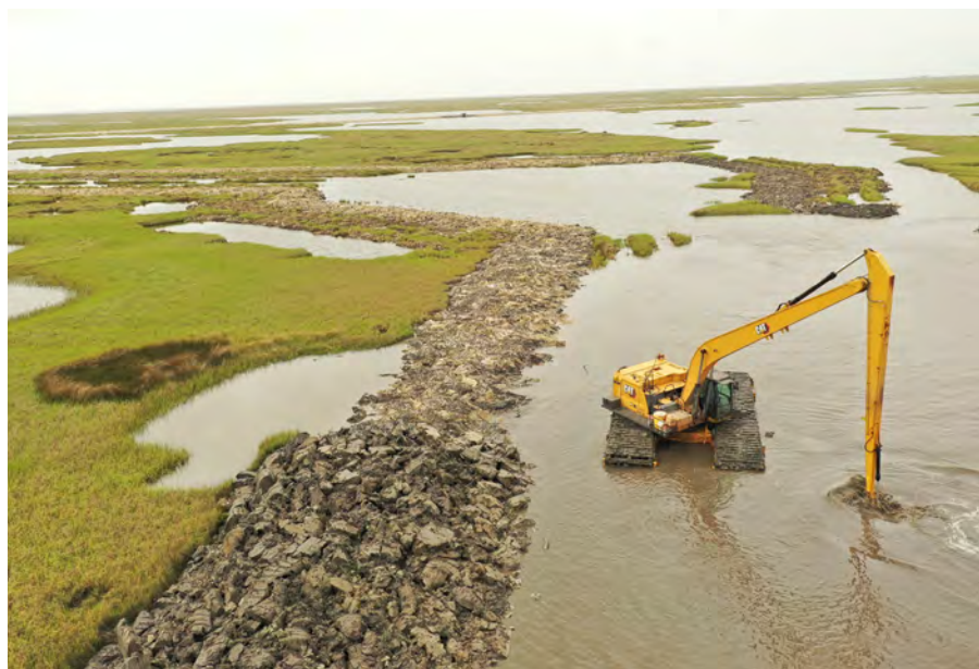
Marsh platforms under construction at Long Point Bayou
