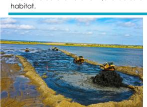
On an average production day, over 40,000 cubic yards of material are pumped through a 30-inch pipe. That's equivalent to over 2,500 double axel dump trucks of sediment being delivered to the project site every day.
