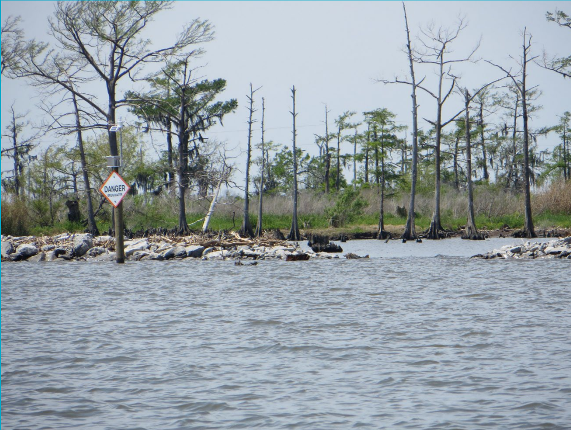
Before: 2013 (Immediately Post-Construction)
