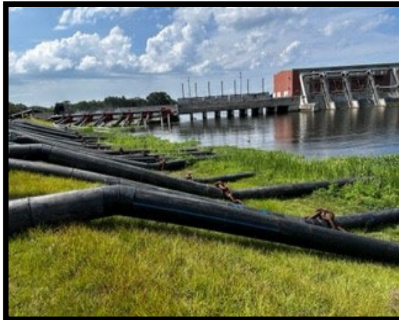
TEMPORARY PUMP PLACEMENT
