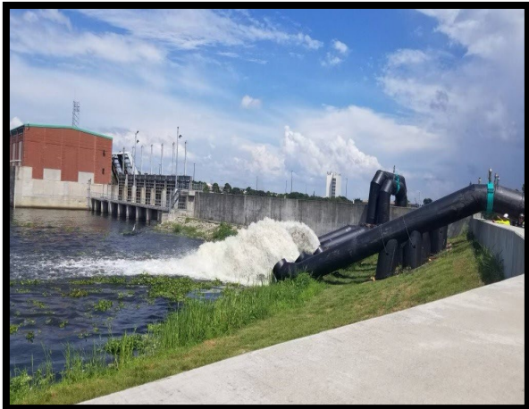
TEMPORARY PUMP PLACEMENT
