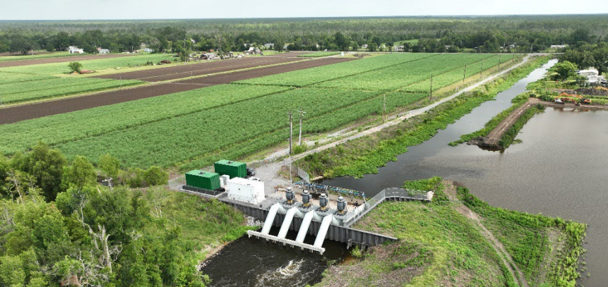
Hanson Canal Pump Station 1,000 CFS Capacity Project Complete & Operational
