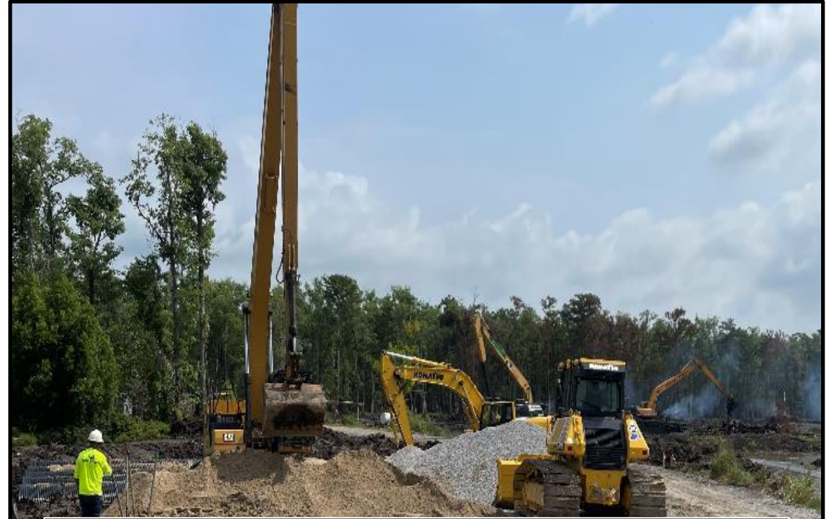
ROW clearing and tree removal/burning at 107
