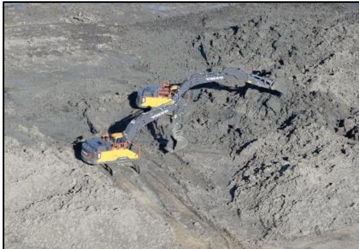
Clay Stockpile 1 on access Road J
