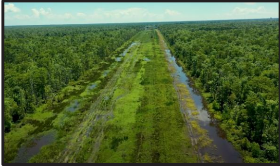
Levees and Floodwalls ($390M Increase)
