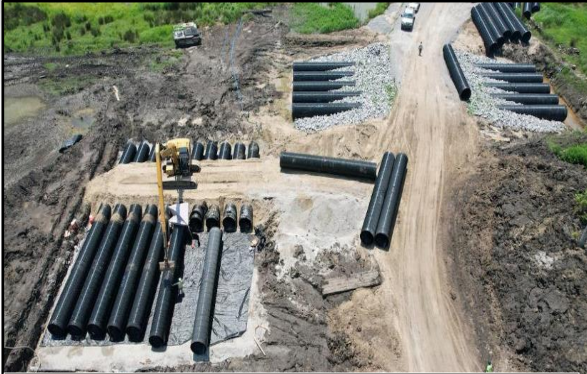
Culvert placement for interior drainage canal at 107
