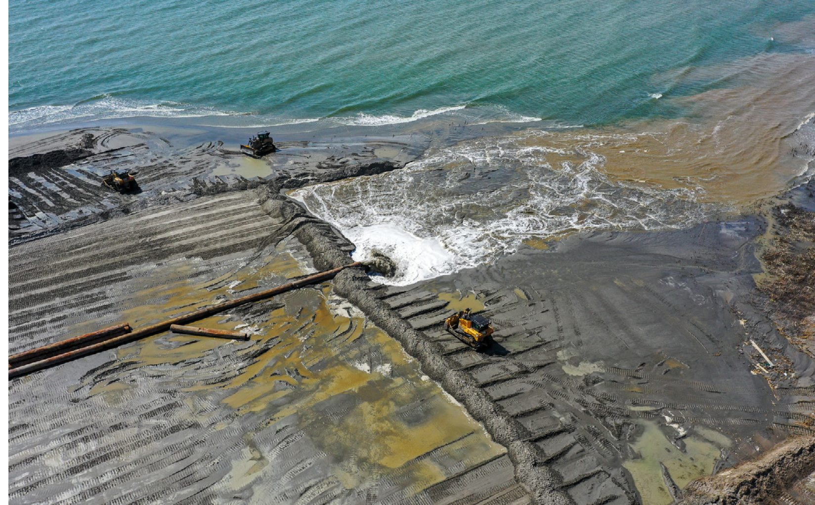
Image: Operations at West Belle Headland after Hurricane Ida, 2021 (CPRA)
