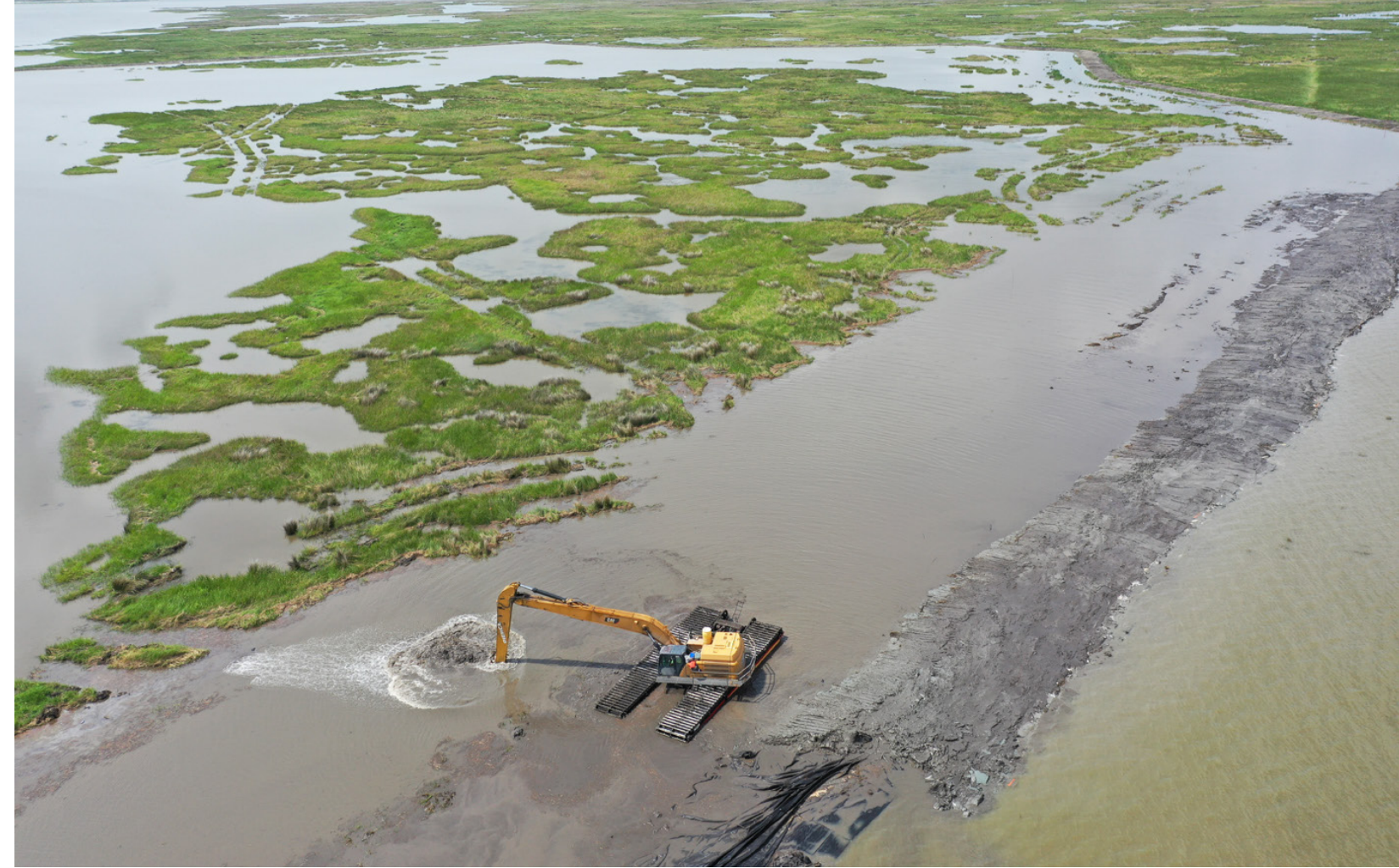
Image: Marsh Creation construction of the New Orleans Landbridge, 2022 (CPRA)
