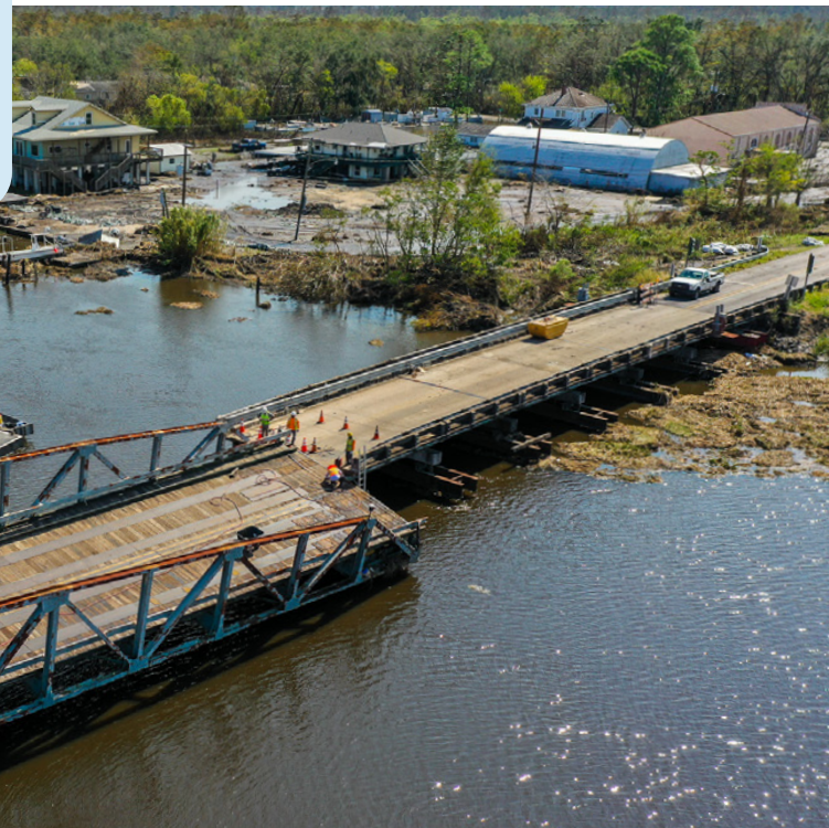
Image: Bridge Repair Post Hurricane Ida, Lafitte, 2021 (CPRA)
