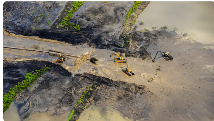
Image: Project Construction (Lindsey Janies)
