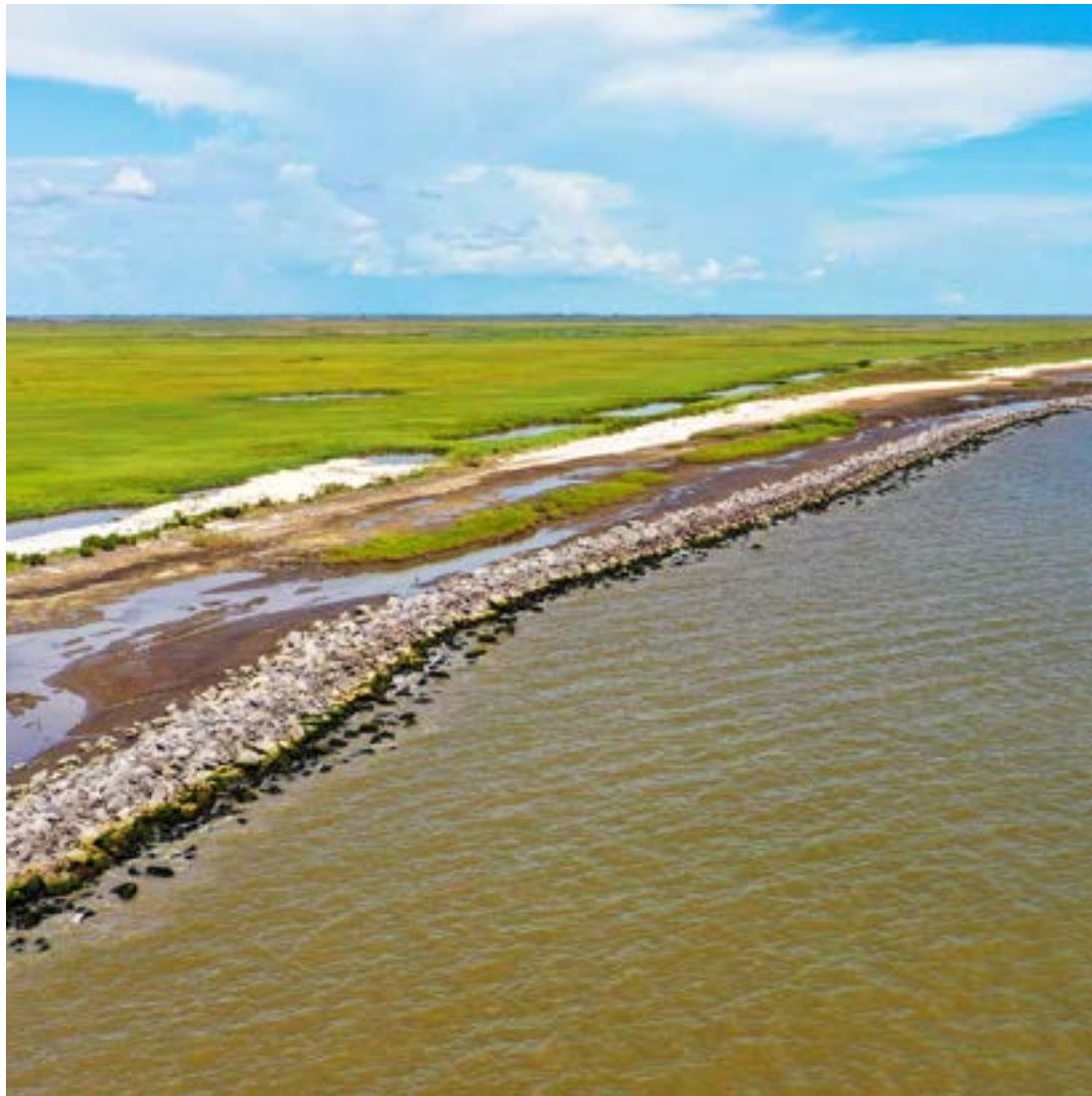
Current breakwaters along the shoreline of Cameron Parish
