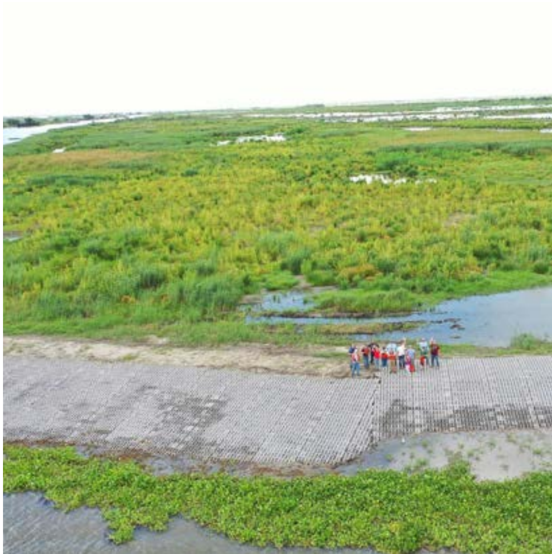
CPRA team members standing on newly constructed concrete mats
