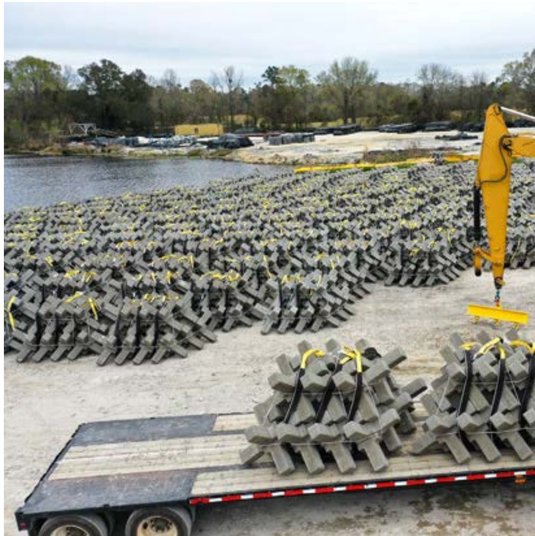
Concrete ShoreJax being delivered for project construction
