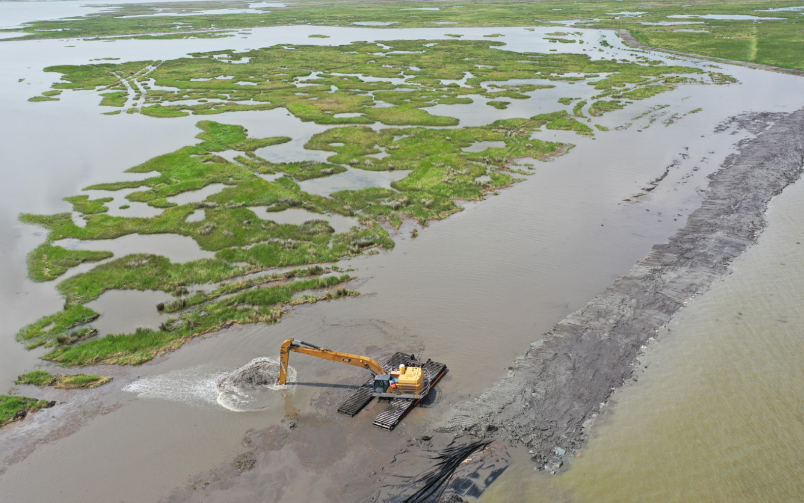
Image: Marsh Creation construction of the New Orleans Landbridge, 2022 (CPRA)
