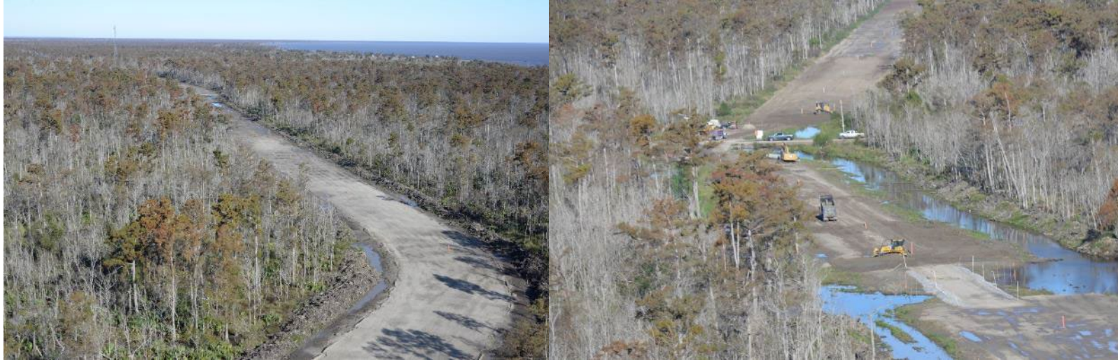
SP2 Sand base placed along levee alignment
