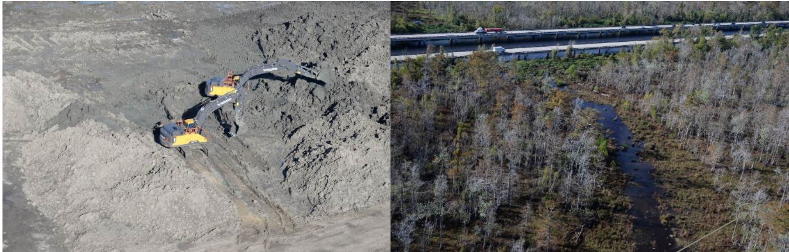
Clay Stockpile 1 on access Road J
