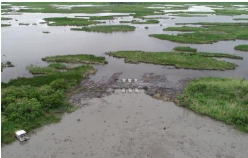
3 WCS, 4 breach repairs, and rock riprap
