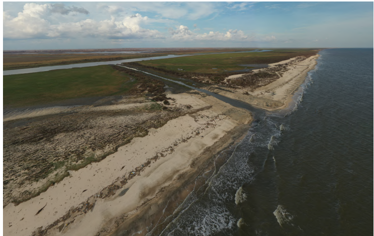
Completed Mermentau Cut in Cameron Parish
