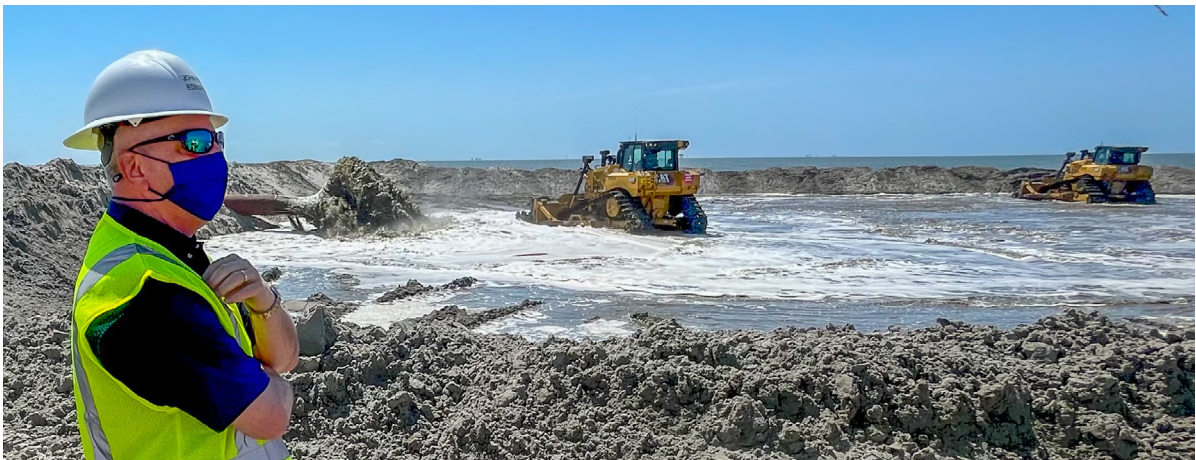
Gov. John Bel Edwards visits Trinity-East Island during restoration
