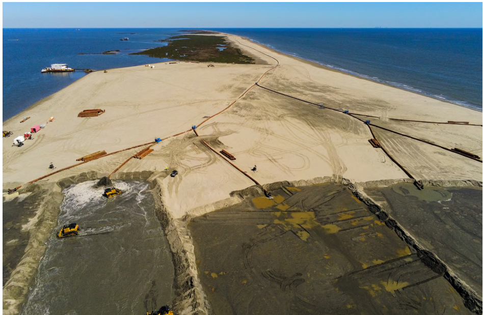
Before and After Terrebonne Basin Barrier Island Restoration
