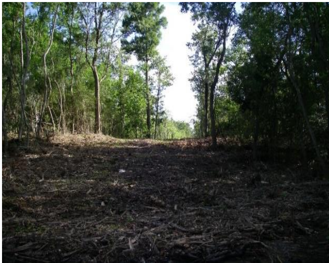
Example of spoil bank adjacent to pipeline.
