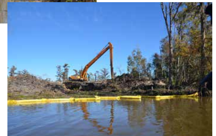
Channels dredged through the spoil bank levee not only help drain the swamp, but also allows the periodic flow of fresh river water and nutrients into the swamp basin.
