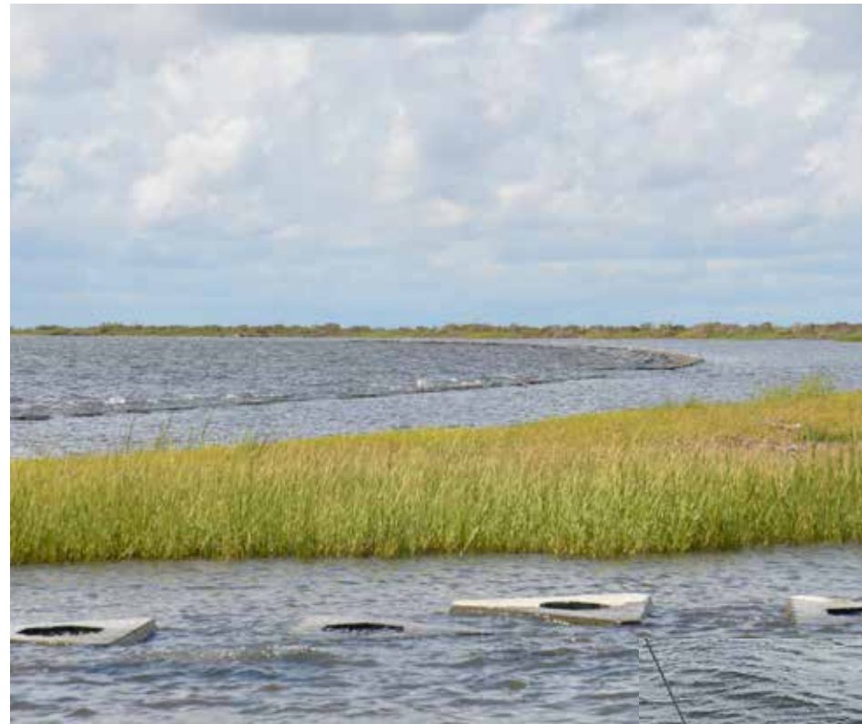
Workers place one of the four types of artificial reef structures designed to attenuate wave action, increase biodiversity along with oyster development, and allow sediment accretion between the shore and the reef.
