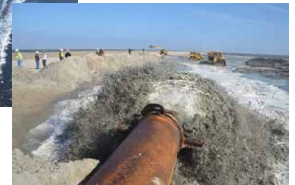
To restore the 13 miles of headland, CPRA used more than 8.4 million cubic yards of sand to create 1059 acres of beach and dune, roughly an area equivalent of almost 1047 football fields.
