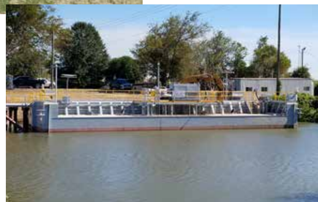
When conditions make it necessary, this barge gate at Lockport can be closed to prevent the progression of saltwater up Bayou Lafourche.
