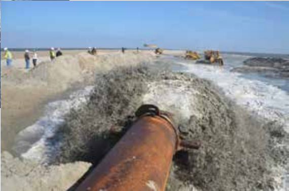
To restore the 13 miles of headland, CPRA used more than 8.4 million cubic yards of sand to create 1059 acres of beach and dune, roughly an area equivalent of almost 1047 football fields.
