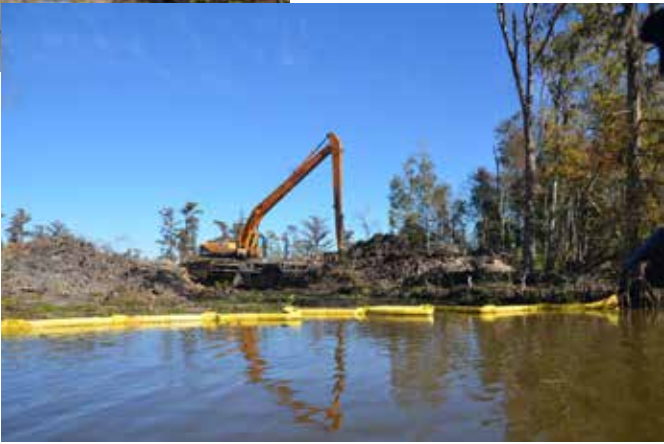
Channels dredged through the spoil bank levee not only help drain the swamp, but also allows the periodic flow of fresh river water and nutrients into the swamp basin.
