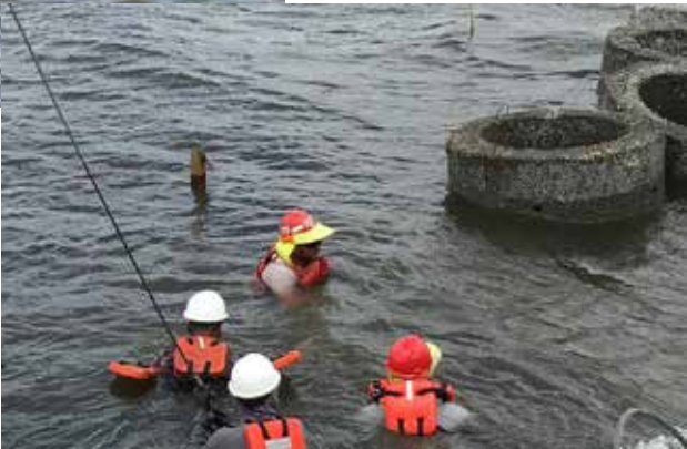
Workers place one of the four types of artificial reef structures designed to attenuate wave action, increase biodiversity along with oyster development, and allow sediment accretion between the shore and the reef.
