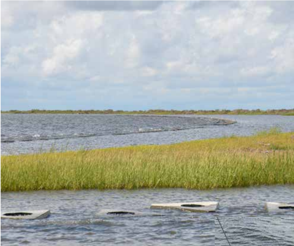
Workers place one of the four types of artificial reef structures designed to attenuate wave action, increase biodiversity along with oyster development, and allow sediment accretion between the shore and the reef.
