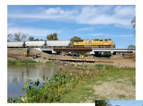
Culverts under the old railroad bridge restricted the amount of water that could be pumped from the Mississippi River at Donaldsonville. CPRA helped fund the construction of a new open span bridge that now allows the pumps (also funded by CPRA) to send more fresh water down Bayou Lafourche.
