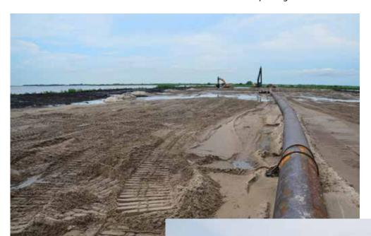
All of this brown "dirt" is actually sediment dredged from the bottom of the nearby Mississippi River and pumped through more than 13 miles of pipeline to its final destination, turning open water areas into land and marsh.
