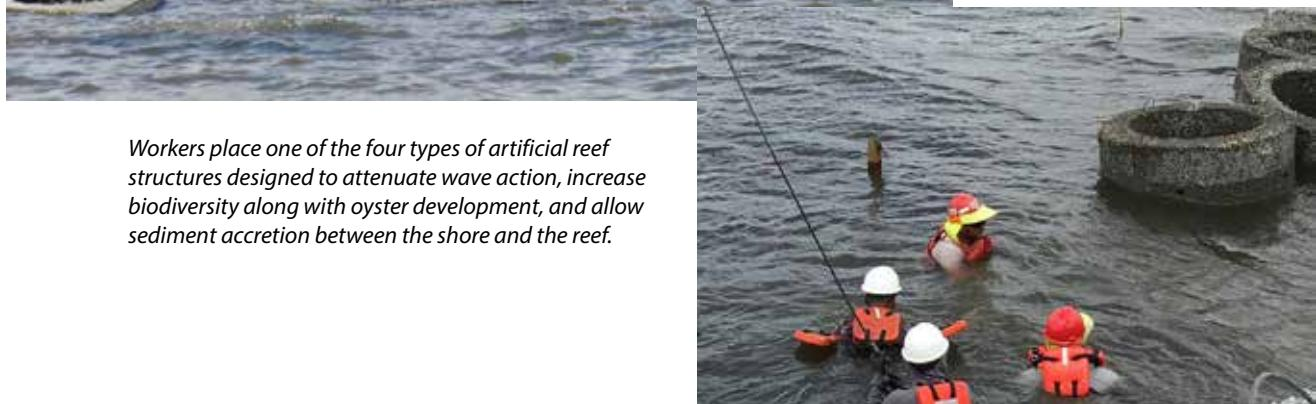
*Workers place one of the four types of artificial reef structures designed to attenuate wave action, increase biodiversity along with oyster development, and allow sediment accretion between the shore and the reef.*
