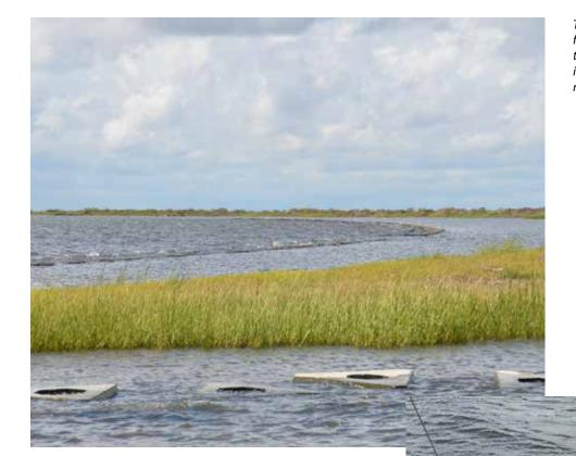
The calming effect of even a small foreshore barrier is evident as the energy of the choppy water is dissipated before reaching the marsh edge.
