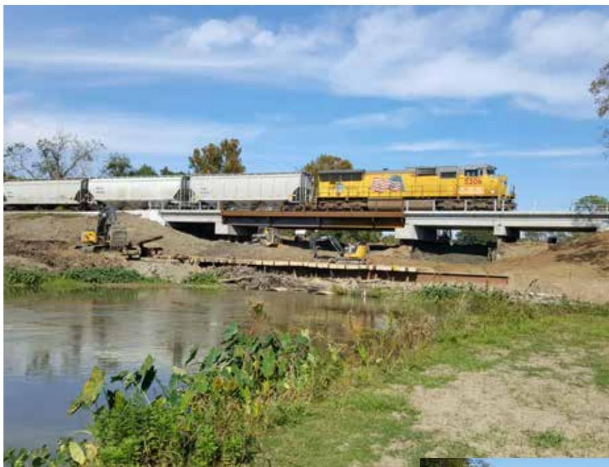
*Culverts under the old railroad bridge restricted the amount of water that could be pumped from the Mississippi River at Donaldsonville. CPRA helped fund the construction of a new open span bridge that now allows the pumps (also funded by CPRA) to send more fresh water down Bayou Lafourche.*
