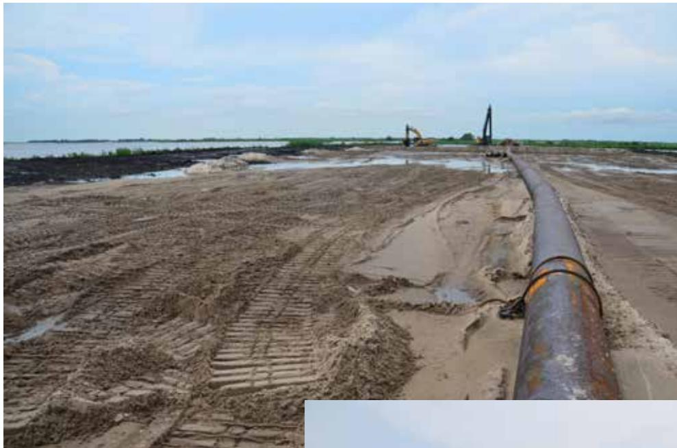
*All of this brown "dirt" is actually sediment dredged from the bottom of the nearby Mississippi River and pumped through more than 13 miles of pipeline to its final destination, turning open water areas into land and marsh.*
