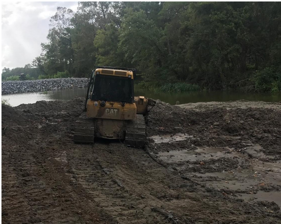
Grading of newly dredged and placed material within the canal.
