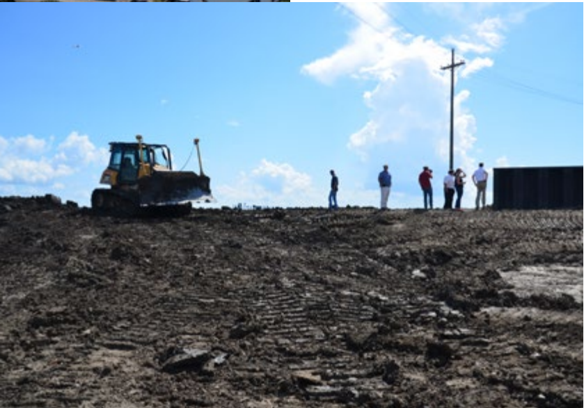
Built in two increments, the levee totals more than 4.3 miles in length along Falgout Canal Road between Bayou Dularge Road and the Houma Navigation Canal. Built to a height of 12 feet, it will settle into its design height of 10 feet to achieve a protection level of 25 years.
