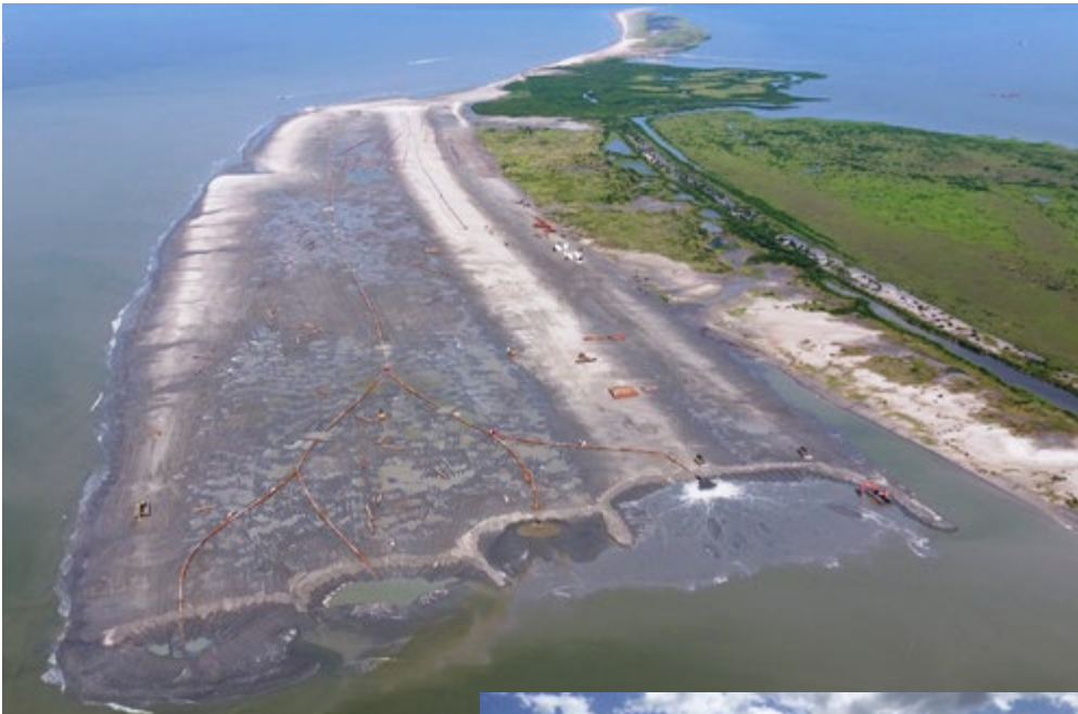
Approximately 10.4 million cubic yards of dredged material was pipelined from a borrow area nine miles offshore to restore more than 900 acres of barrier island and marsh habitat. The project was paid for with funds from the Deepwater Horizon Natural Resources Damage Assessment (NRDA) Early Restoration Program.
