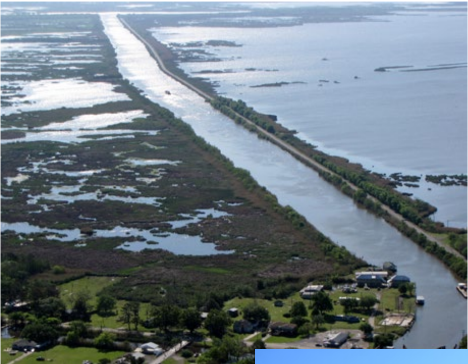
Built in two increments, the levee totals more than 4.3 miles in length along Falgout Canal Road between Bayou Dularge Road and the Houma Navigation Canal. Built to a height of 12 feet, it will settle into its design height of 10 feet to achieve a protection level of 25 years.
