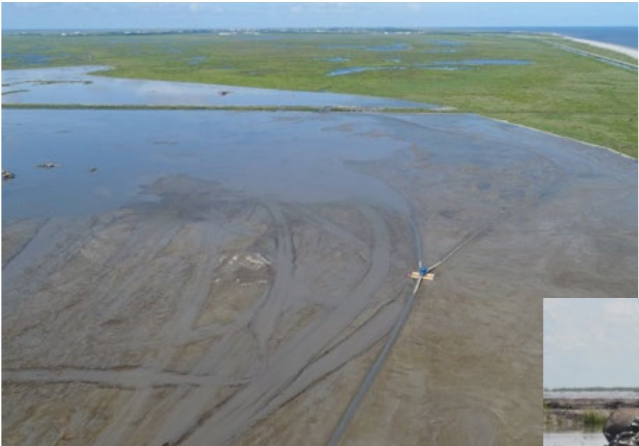
Creating a marsh habitat involves more than just filling an area with sediment. This ecosystem will benefit from the elements planned and achieved prior to the pumping of offshore fill material. Tidal creeks and ponds were constructed and retention levees were strategically gapped to achieve a functional marsh that supports estuarine fisheries' access.
