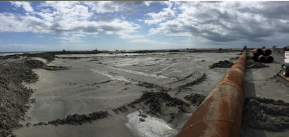
Approximately 10.4 million cubic yards of dredged material was pipelined from a borrow area nine miles offshore to restore more than 900 acres of barrier island and marsh habitat. The project was paid for with funds from the Deepwater Horizon Natural Resources Damage Assessment (NRDA) Early Restoration Program.
