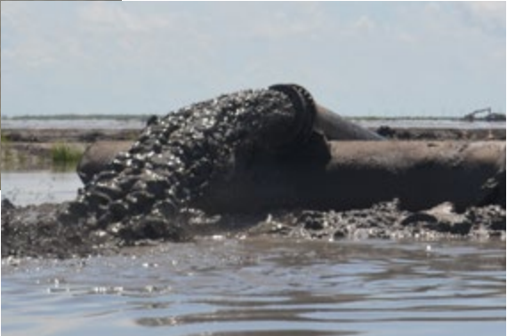
Creating a marsh habitat involves more than just filling an area with sediment. This ecosystem will benefit from the elements planned and achieved prior to the pumping of offshore fill material. Tidal creeks and ponds were constructed and retention levees were strategically gapped to achieve a functional marsh that supports estuarine fisheries' access.
