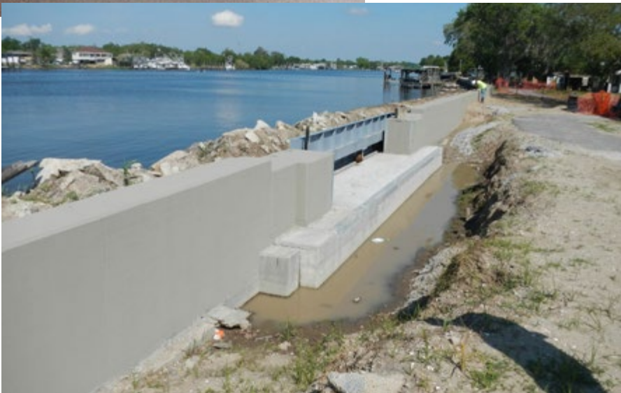
The three miles of floodwalls and earthen levee improvements include six swing gates and five roller gates that can be closed during expected high tides and storm surges.
