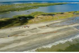
Photos courtesy of Patrick M. Quigley and Lindsey Janies Photography Top: Long Distance Sediment Pipeline Corridor; Bottom: Caminada Headland Beach and Dune Restoration - Aerial images of barrier shoreline restoration efforts along the Caminada shoreline
