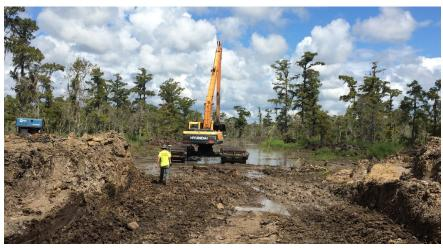
Hydrologic Restoration of the Amite River Diversion Canal (ARDC) (PO-0142): The top image shows a view of a partial cut through the ARDC dike. The cleared channel is visible in the background. The bottom image shows a view of the cleared channel prior to opening of the ARDC dike. Note impounded water in the swamp due to the ARDC dike.
