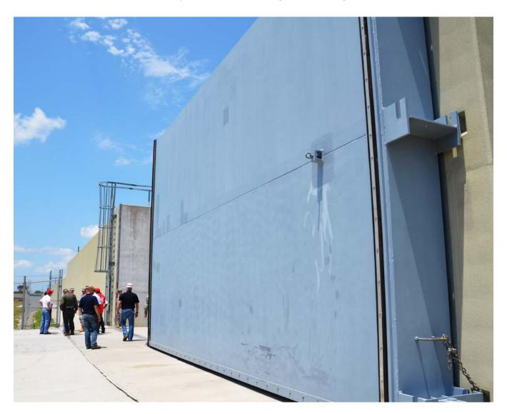
Engineers with the U.S. Army Corps of Engineers inspect one of the massive flood gates in the \$1.4 billion hurricane protection system on the West Bank of greater metropolitan New Orleans. When the system is completely closed the city could still flood from torrential rains, so 75 pump stations—including the world's largest pump station—have been installed for water removal.
