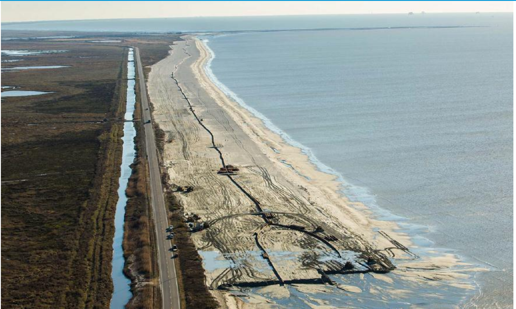
Active project site looking east toward Calcasieu Ship Channel (jetties visible in background). Vegetation line on landward edge of beach represents the pre-construction shoreline location.
