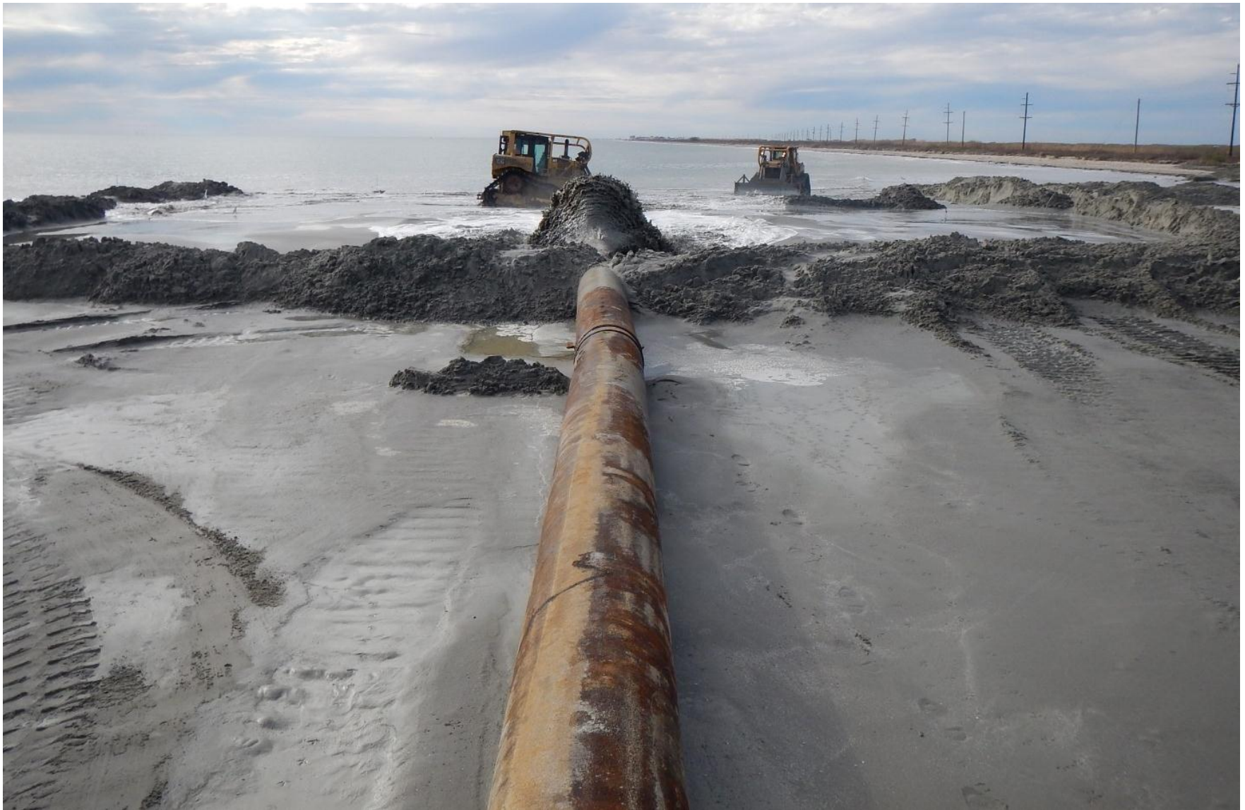
Slurry being discharged into template. Training dikes being employed on seaward edge of discharge zone.
