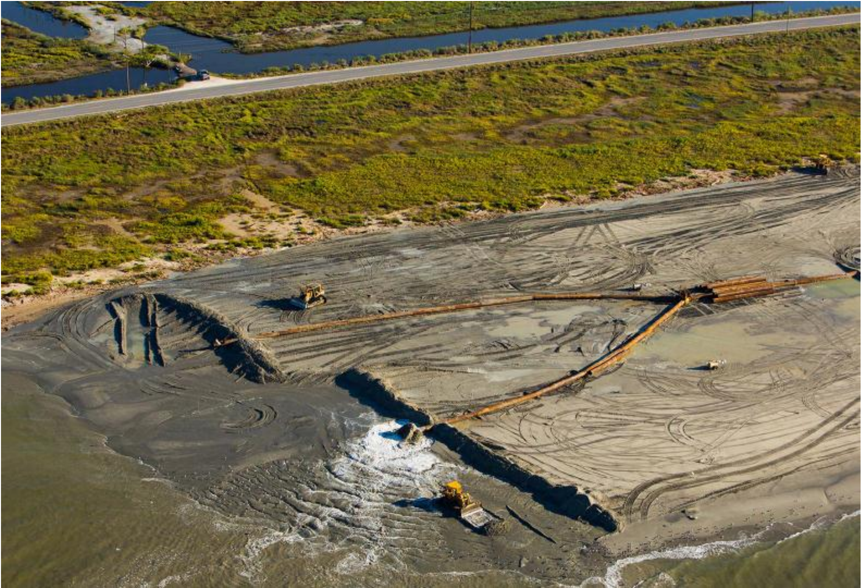
Dozers working sand material being pumped into a 285 ft.-wide beach template
