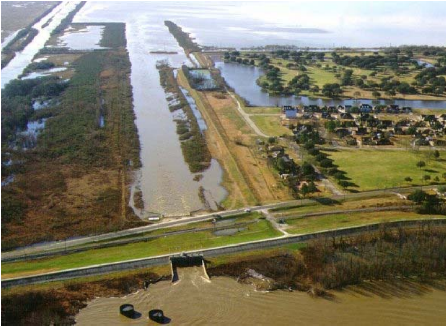
Figure 3.2: The Diversion Structure at Caernarvon (Mississippi River in foreground)
