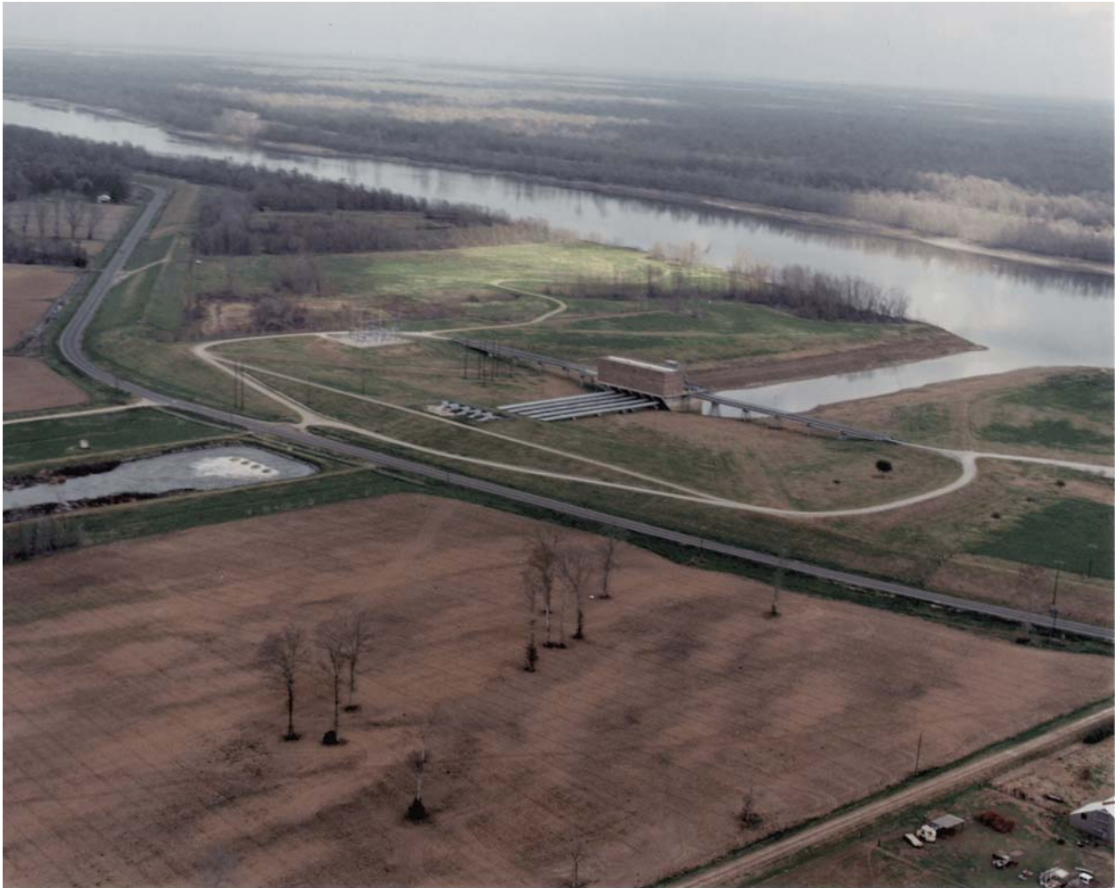
Figure 2.4: Teche/Vermilion Pumping Station
