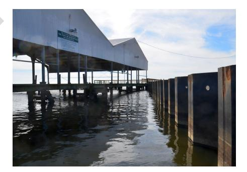
The Franklin Floodgate project constructed a 170-foot steel flood wall, a barge gate, 800 feet of earthen levee, and a large pump house to protect communities, economic centers and critical infrastructure. The project is a partnership between CPRA, OCD-DRU and the St. Mary Parish Levee District.
