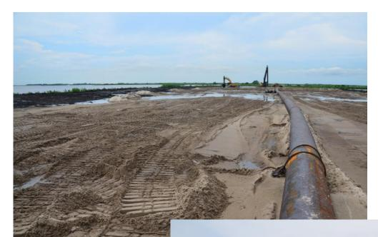
All of this brown "dirt" is actually sediment dredged from the bottom of the nearby Mississippi River and pumped through miles of pipeline to its final destination, turning open water areas into land and marsh.
