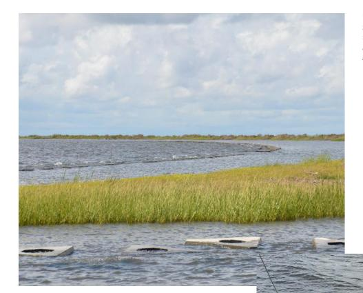
The calming effect of even a small foreshore barrier is evident as the energy of the choppy water is dissipated before reaching the marsh edge.
